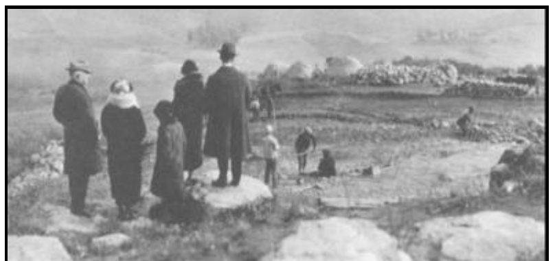
The Fletchers observe the early stages of construction of the Nature Theater.
